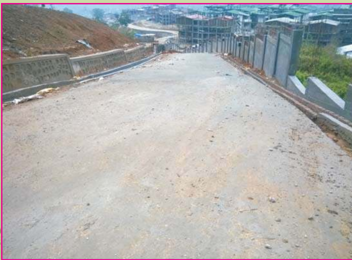
Approach Road to Water Treatment Plant
