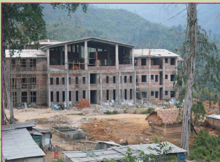
Civil Engineering Block
