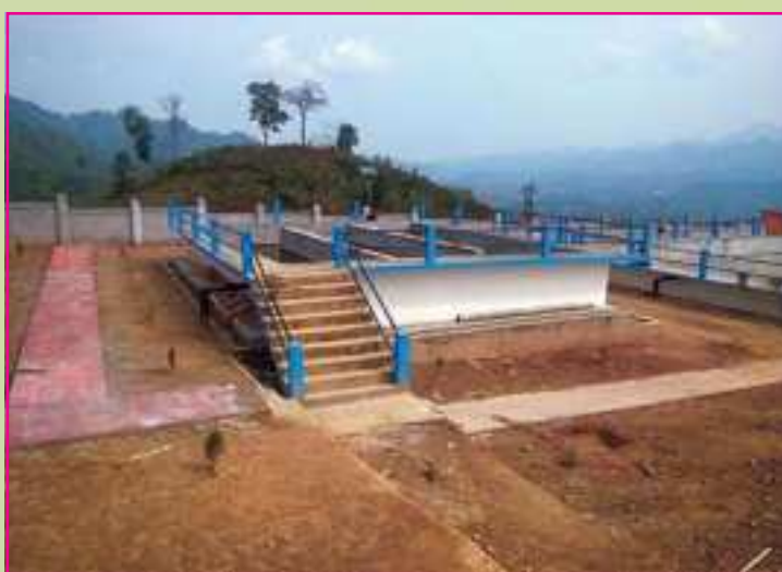
Water Supply System
