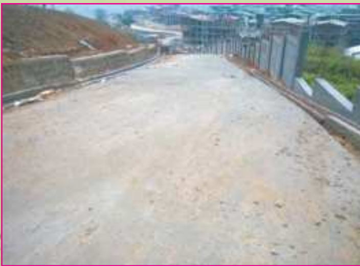
Approach Road to Water Treatment Plant
