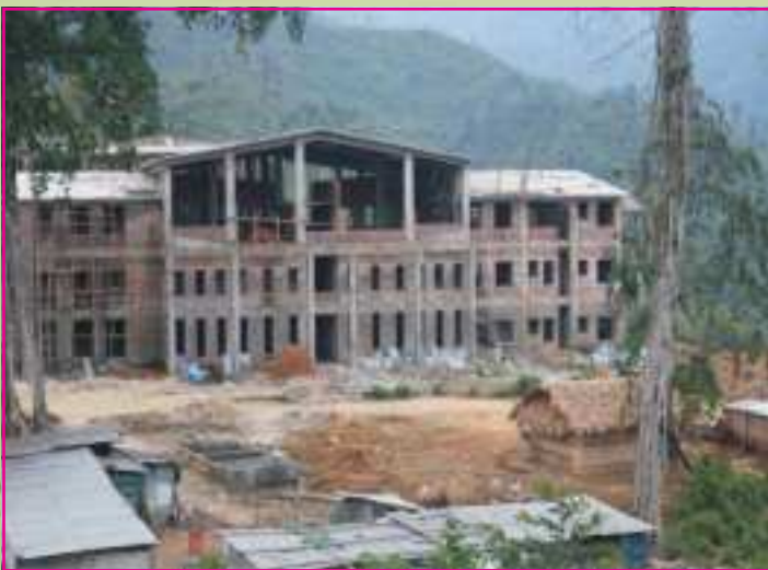
Civil Engineering Block
