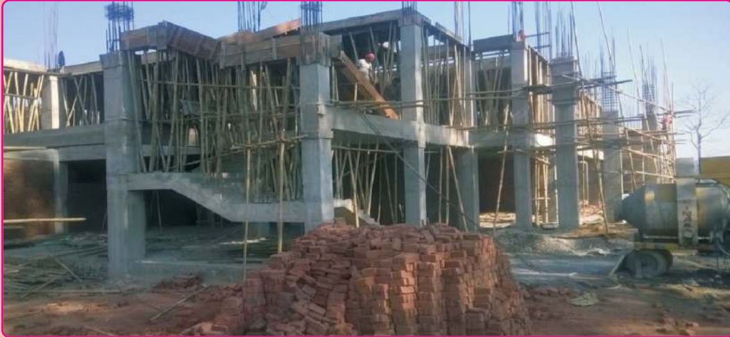
Academic Block: Mechanical Engineering Department.
