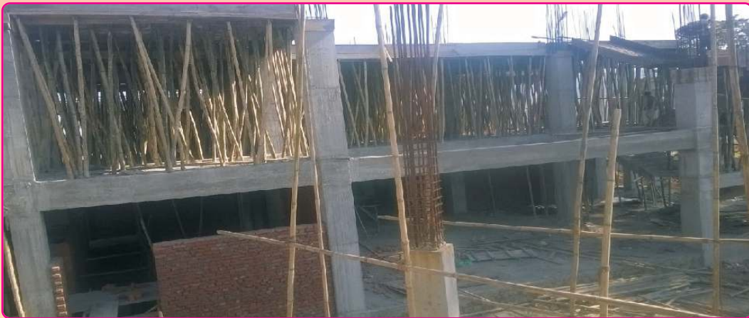
Academic Block: Civil Engineering Department.
