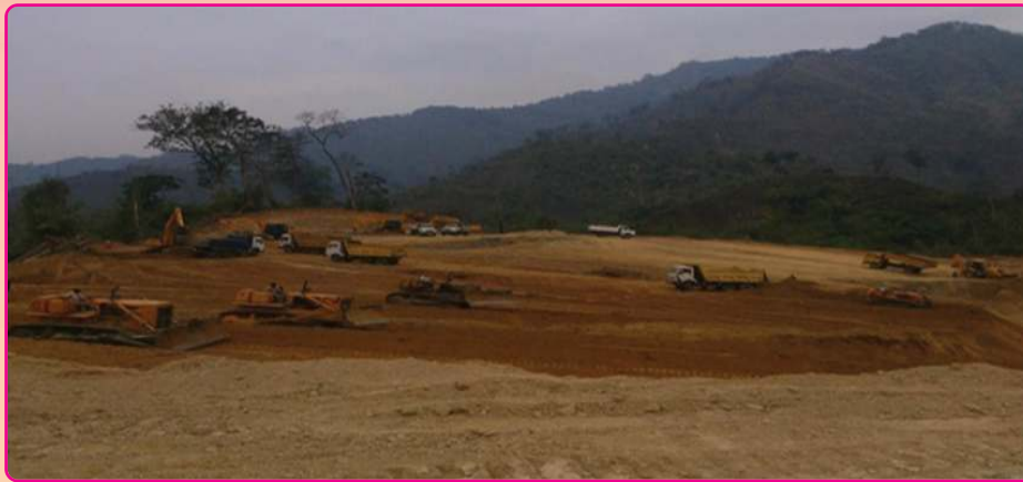
Site after levelling of land
