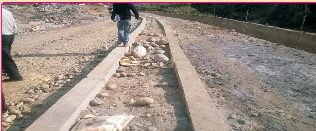
Campus Road and Drain
