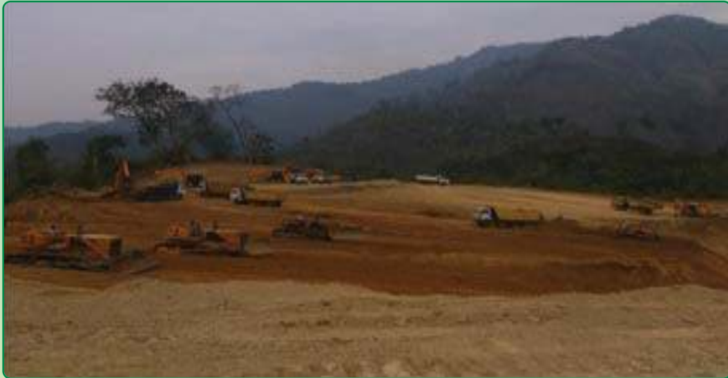
Site after levelling of land
