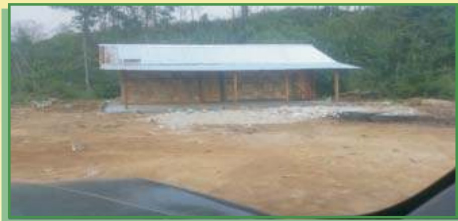
Temporary office-shed for supervising construction works at Jote
