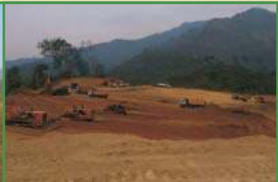
Site after levelling of land
